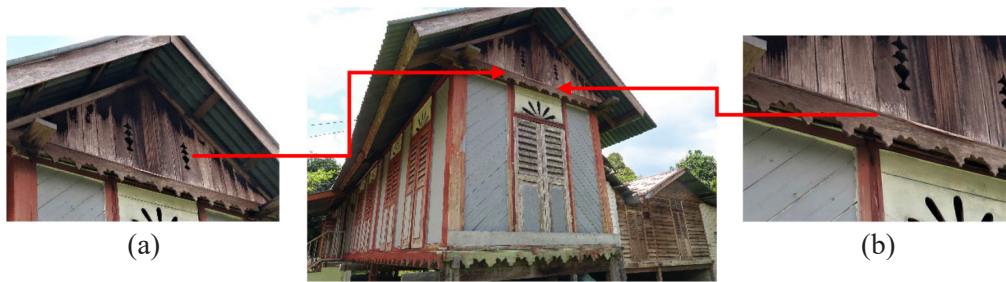
Figure 4: Motifs (a) still-life and (b) fauna on the gable end and fascia board of Ramlah bt. Sulaiman's house.
