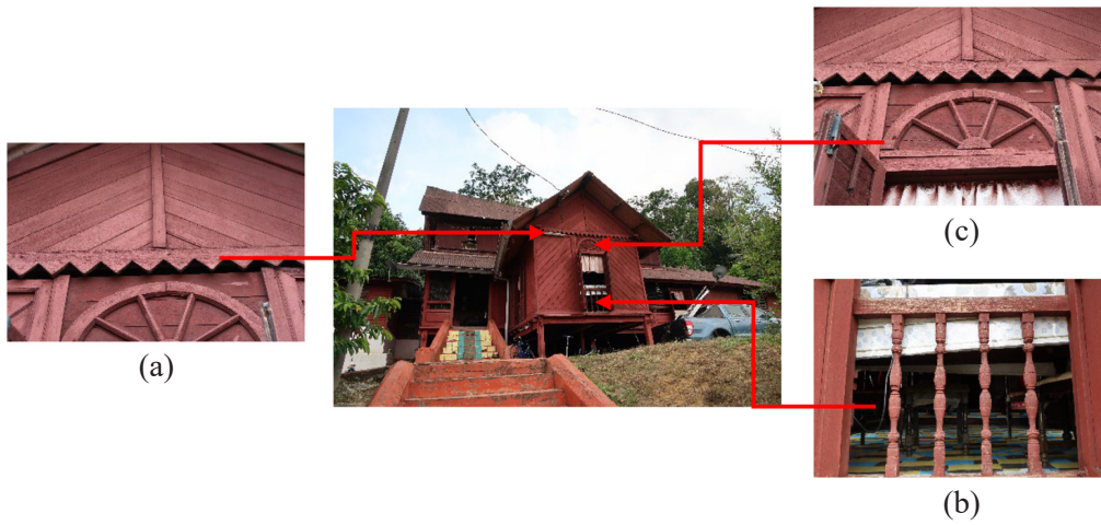
Figure 7: Motifs (a), (b) geometry and (c) cosmos on the fascia board, window head and window rails of Mokhtar Ayub's house.
