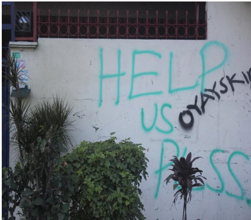
Figure 5: Distress on wall.
